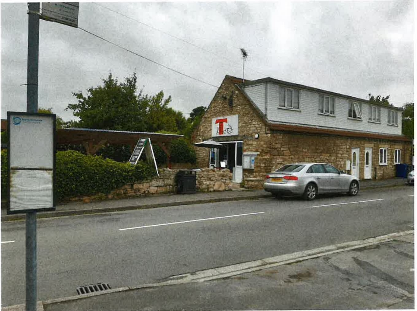
Figure 1 View of premises from the road.
